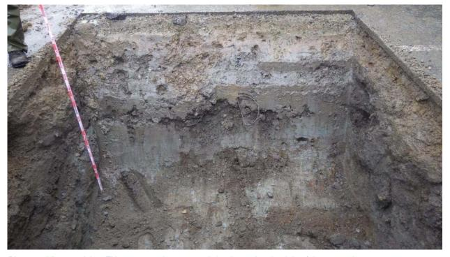
Photo 12: View south into TN-14;-105 and stave-wood pipe located to the right of the measuring tape.
