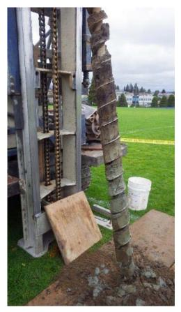
Photo 3: View of matrix in auger at BH16-04, looking northeast.
