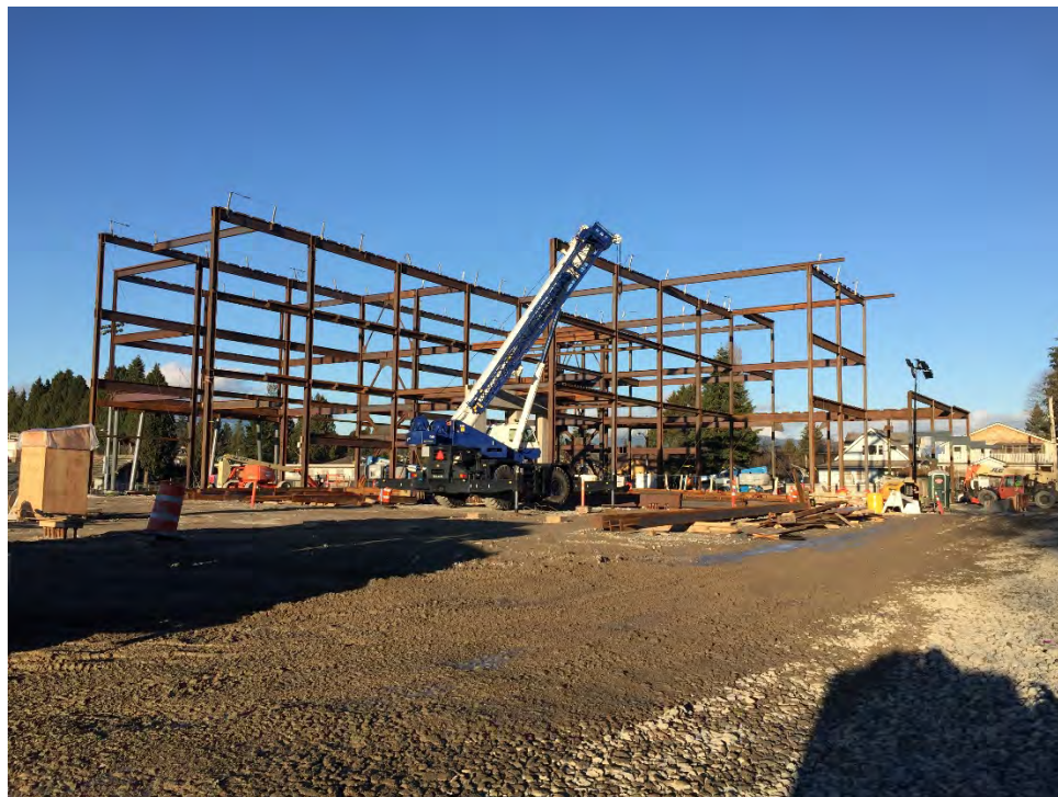
Structural Steel progress as of January 7, 2019
