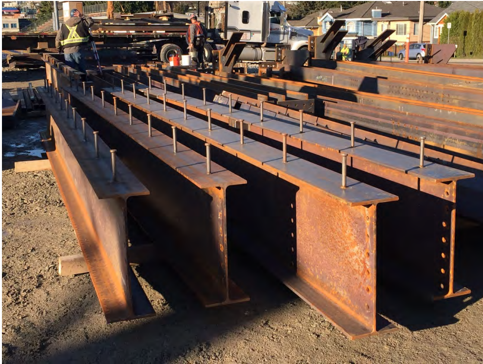
First Structural Steel Arrives on site
