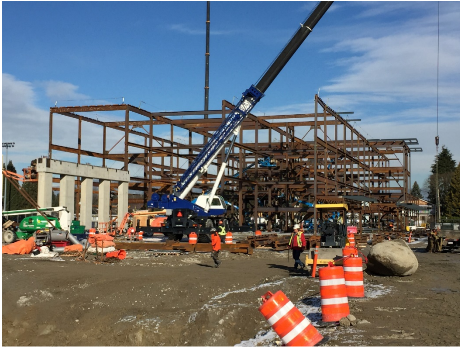
Progress on structural steel
