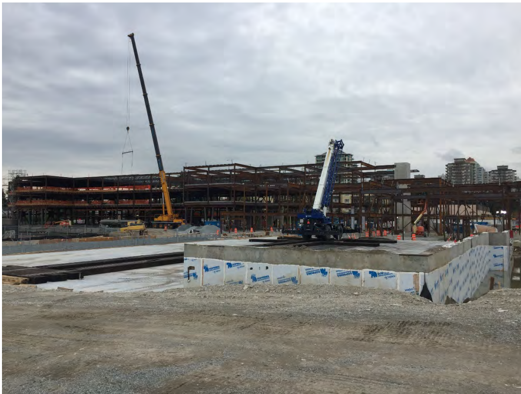
View from gymnasium area
