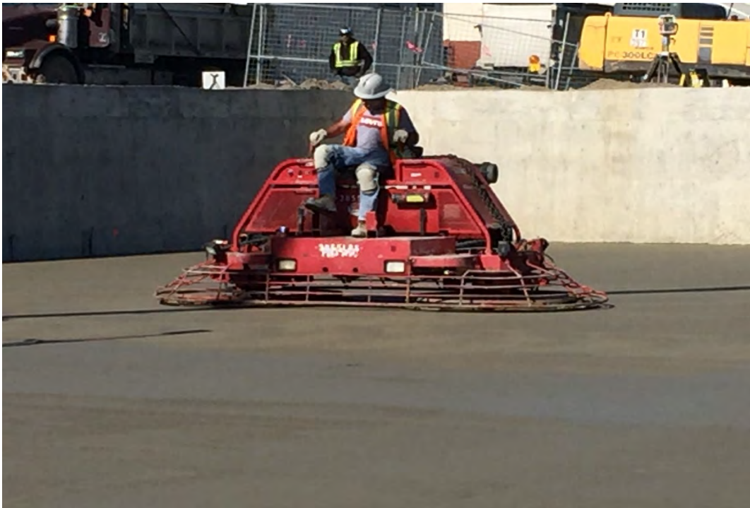
Concrete finishing of gym floor
