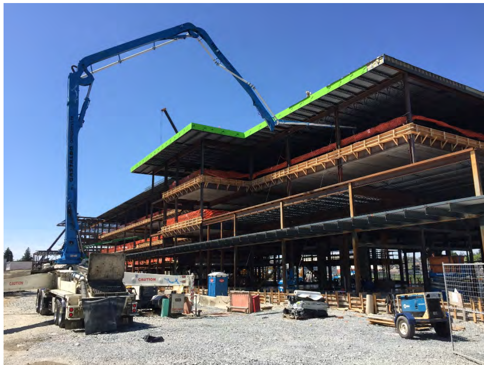
View from 6th Street – Top-lift concrete on 3 rd Floor
