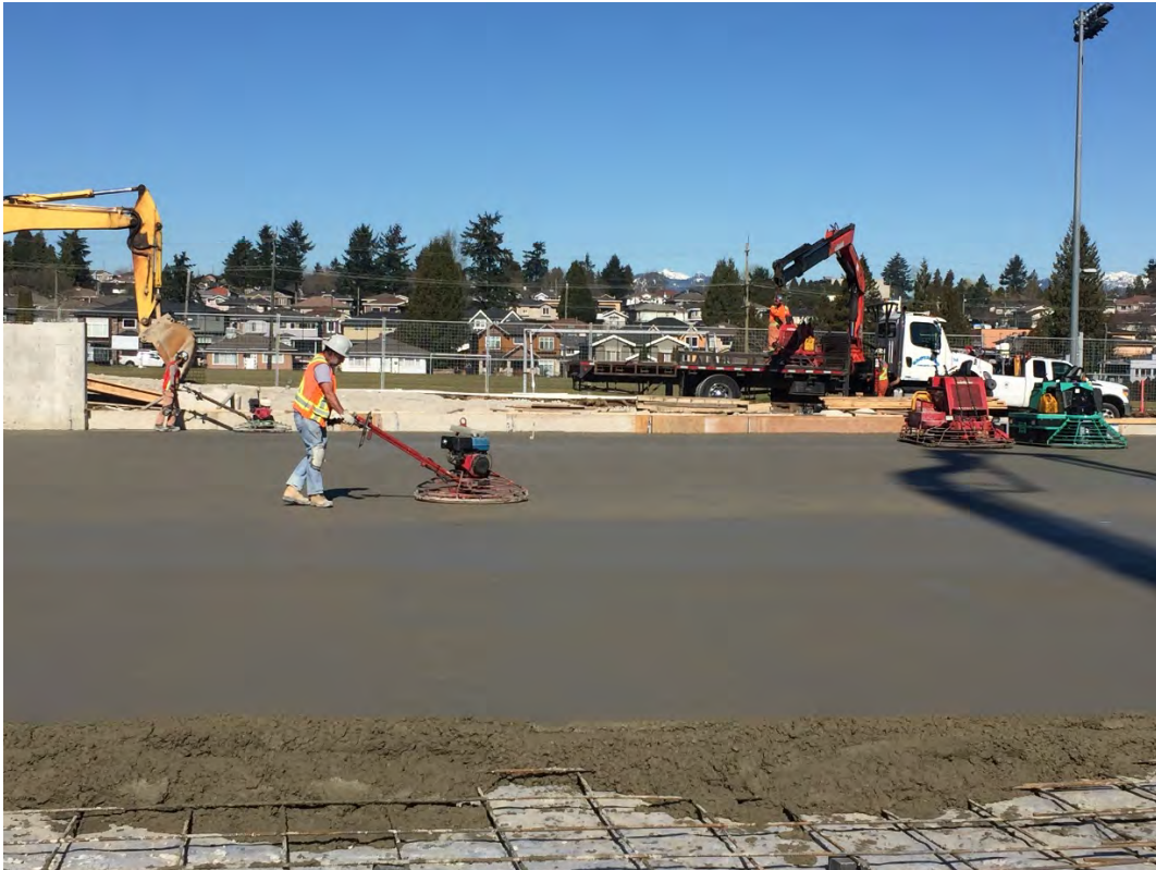
Concrete floor for gymnasium
