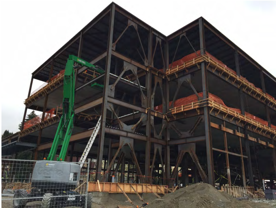
View from 6th Street
