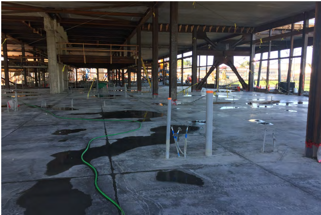
Ground Floor on East Wing facing 6 th Street (CTE Area)
