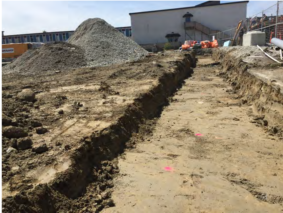
Foundation prep for Maintenance/IT Building
