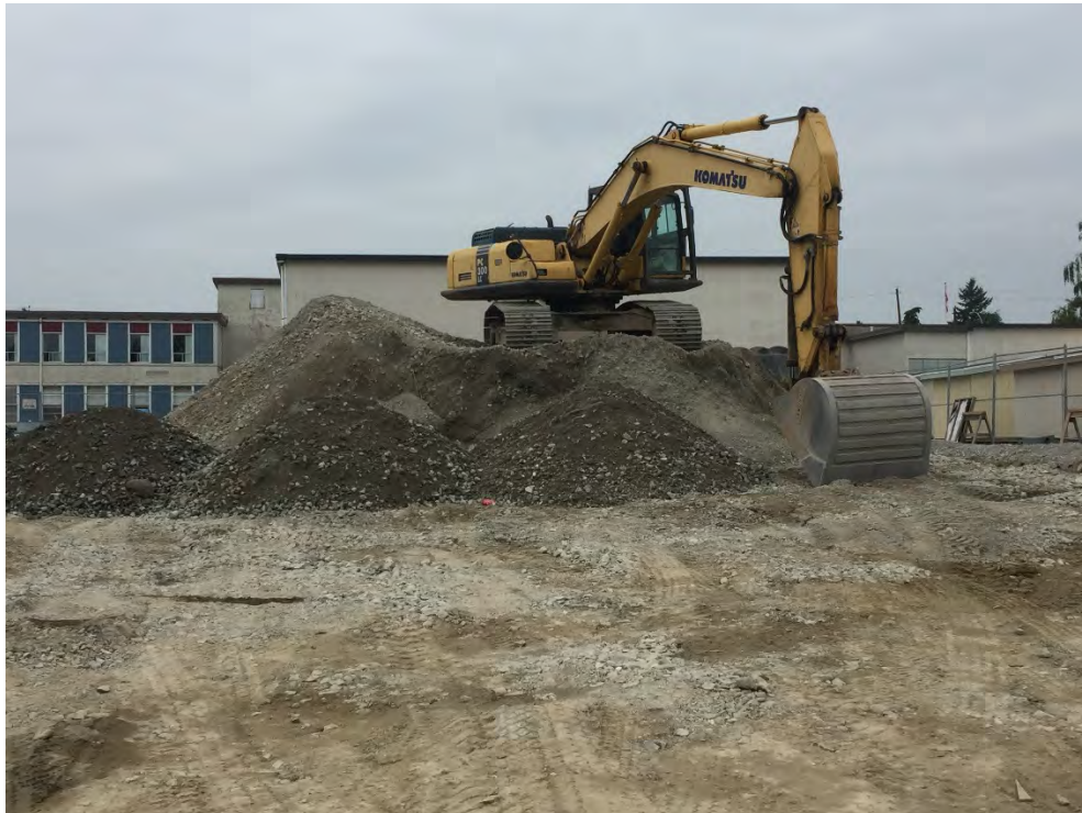
Maintenance/IT Building begins
