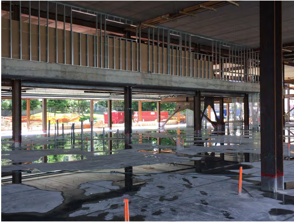
View of Interior and Mezzanine area
