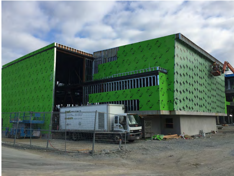
Exterior View by new Theatre
