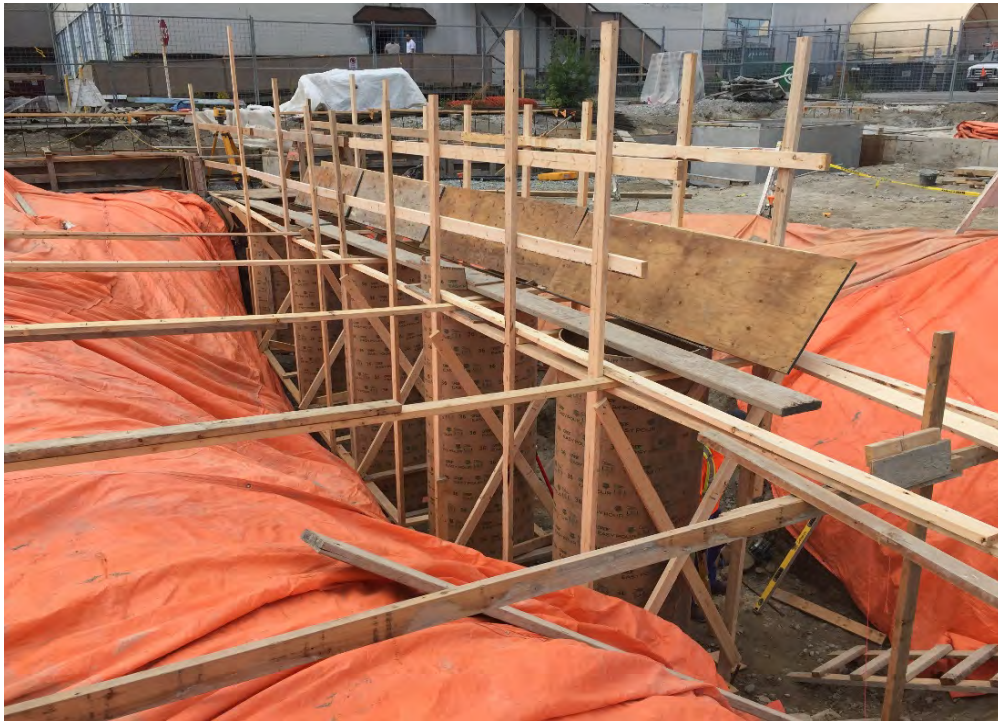
Maintenance/IT Building footings
