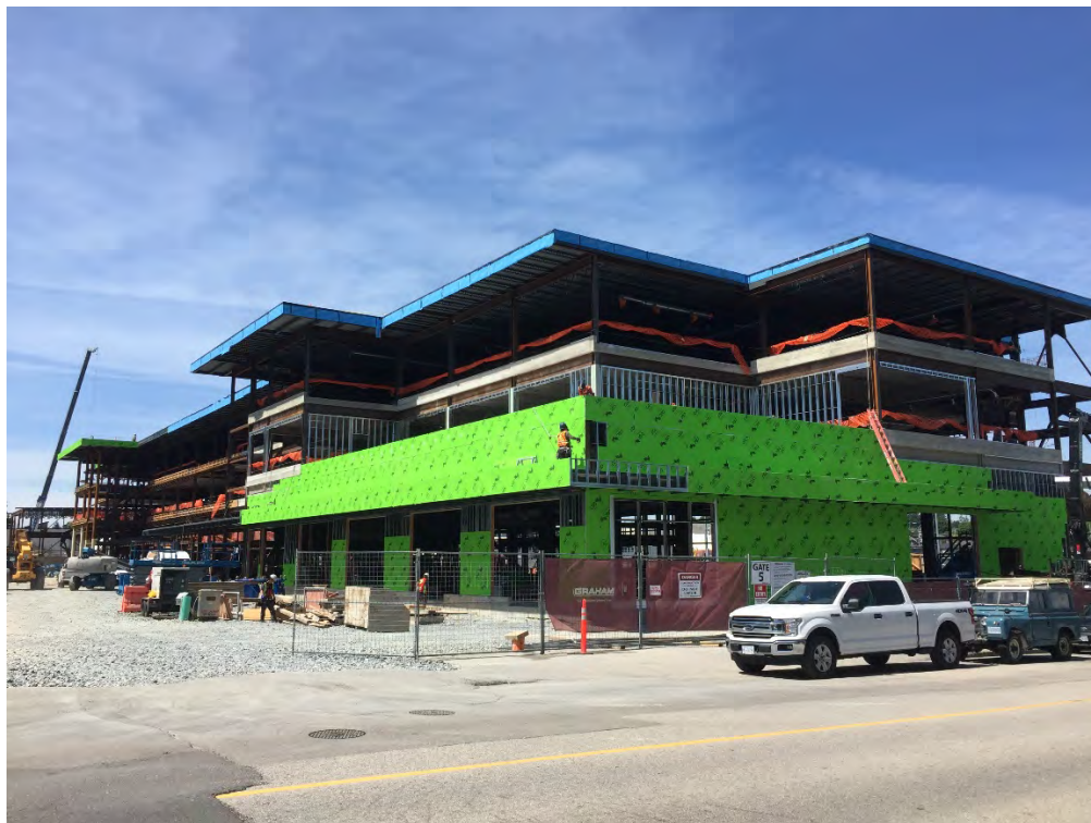
Exterior view from Sixth Street
