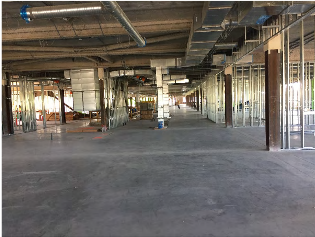
View of Interior and CTE area
