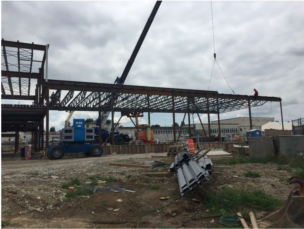
View of Gymnasium
