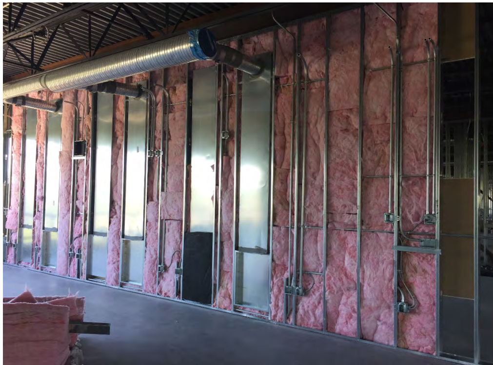
View of 3 rd Floor wall construction.
