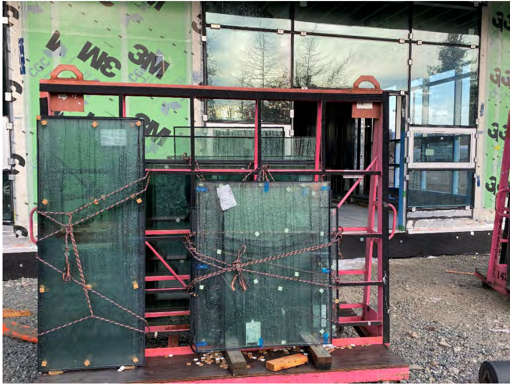
View of Glazing Installation
