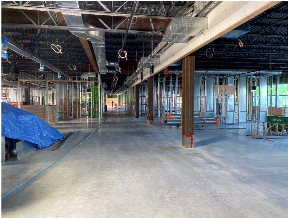
View of 3 rd Floor wall installation
