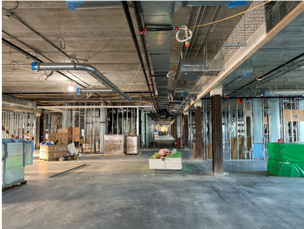
View of Level 2 floor area
