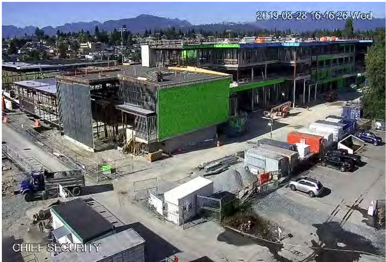
Roof Cam View
