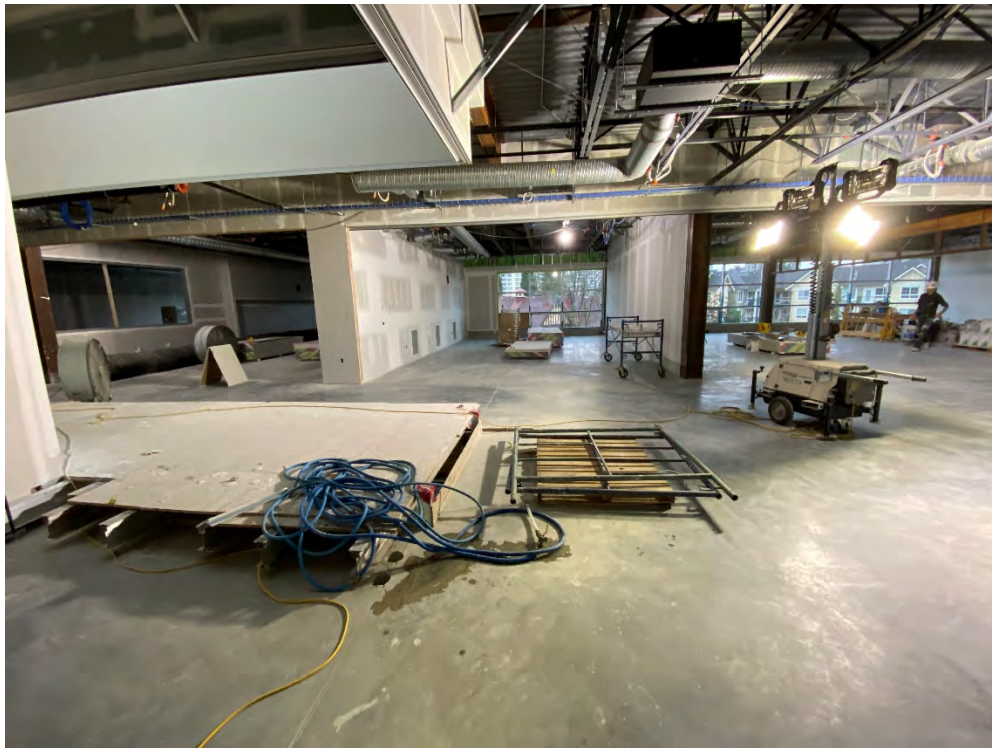
View of Level 2 floor area
