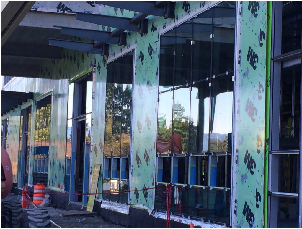
View of Glazing Installation
