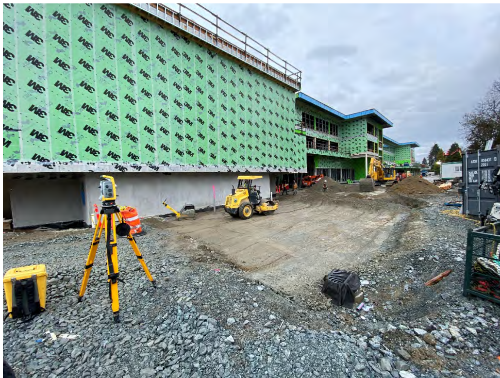
Exterior view from Massey Theatre
