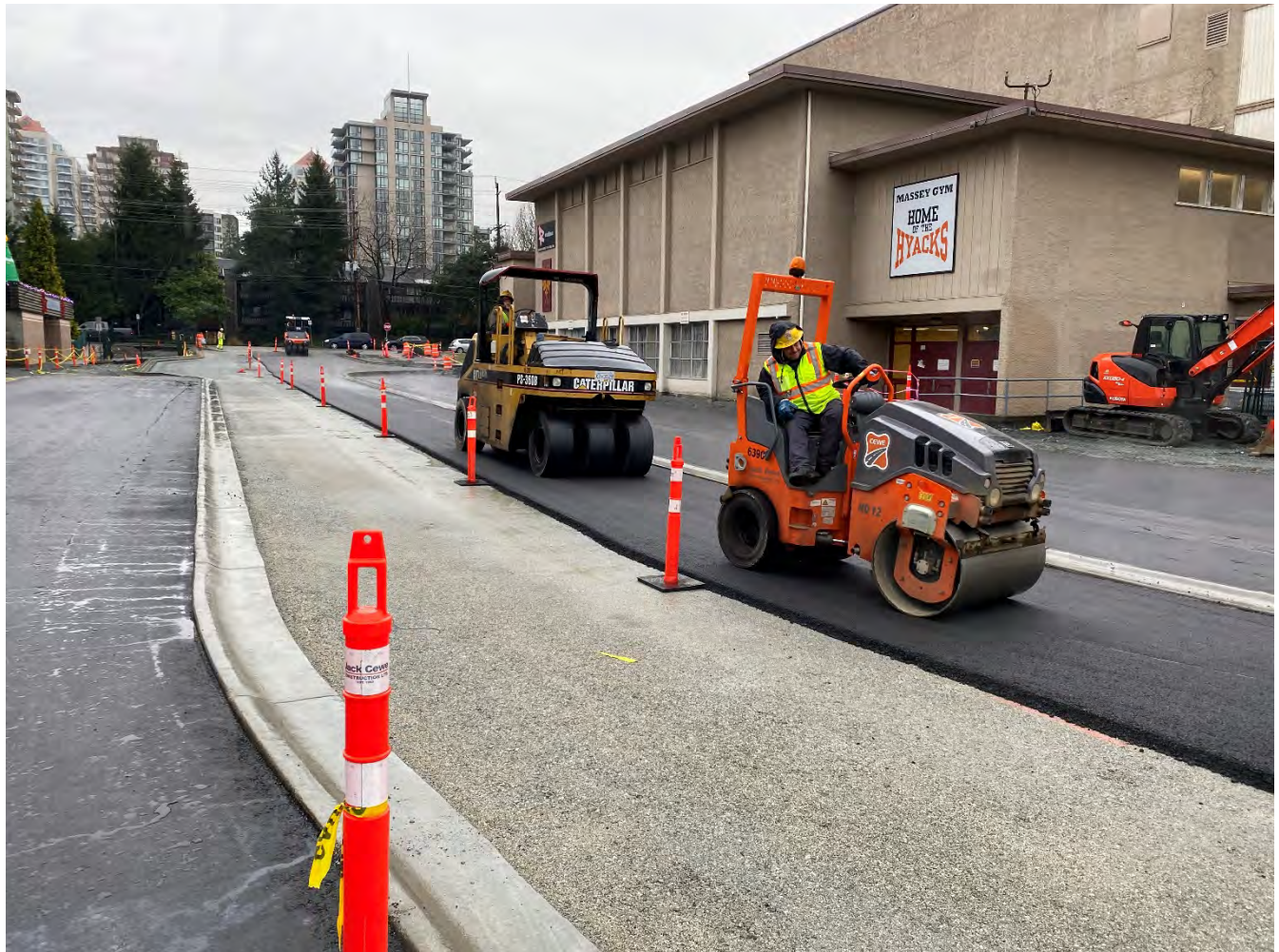
Asphalt Paving on Laneway between Massey Theatre/Moody Park Arena
