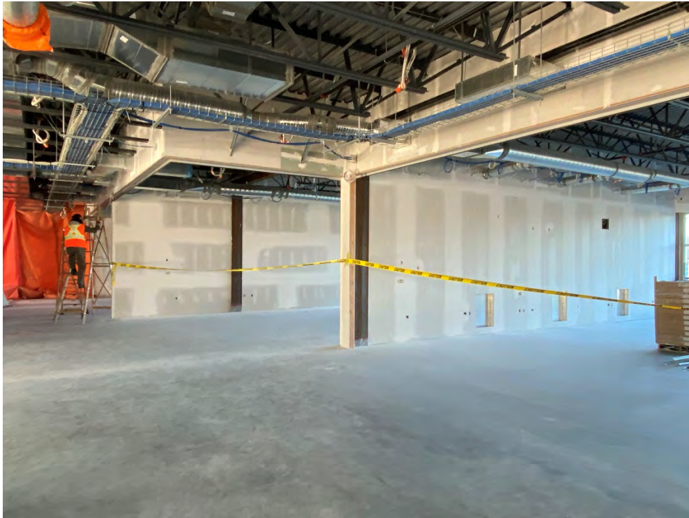
View of 3 rd Floor drywall installation.
