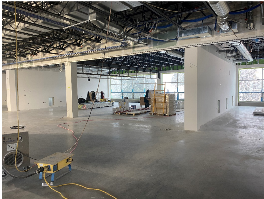
View of Level 2 floor area
