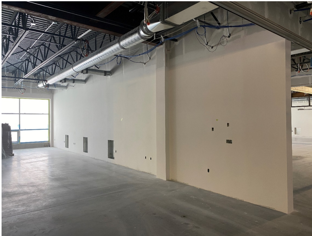
View of 3 rd Floor drywall – painting begins.
