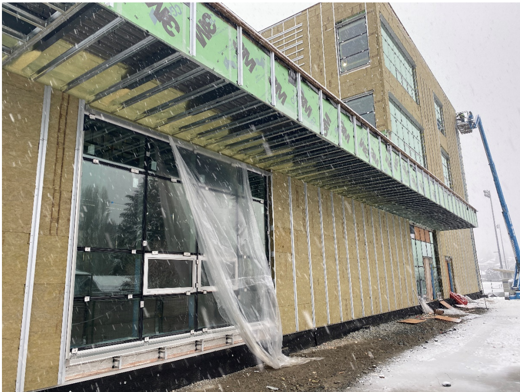
Exterior view from 6 th Street
