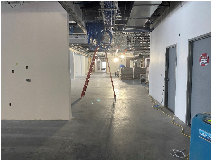
View of 3 rd Floor drywall – painting begins.
