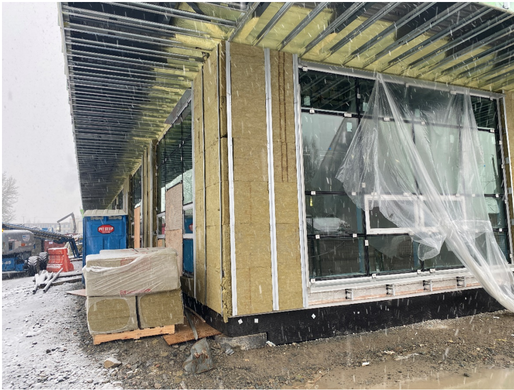
View of Glazing Installation and Insulation
