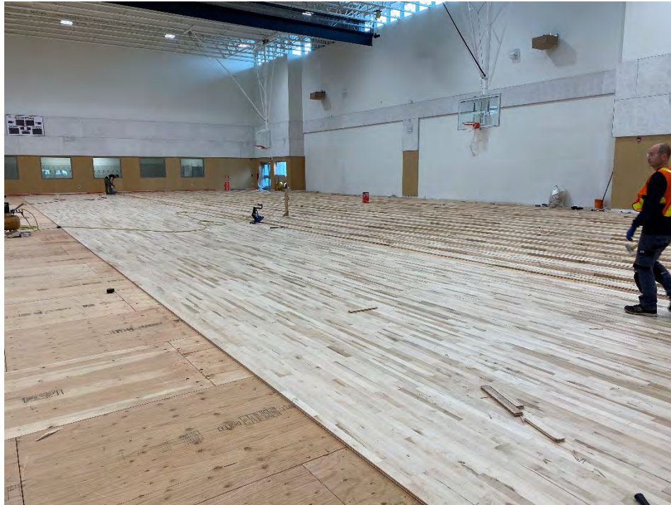
Installation of gymnasium floor
