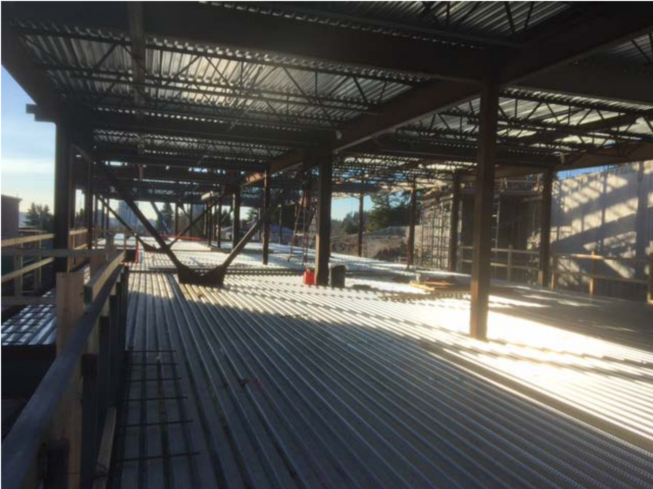
Level 2 decking in progress
