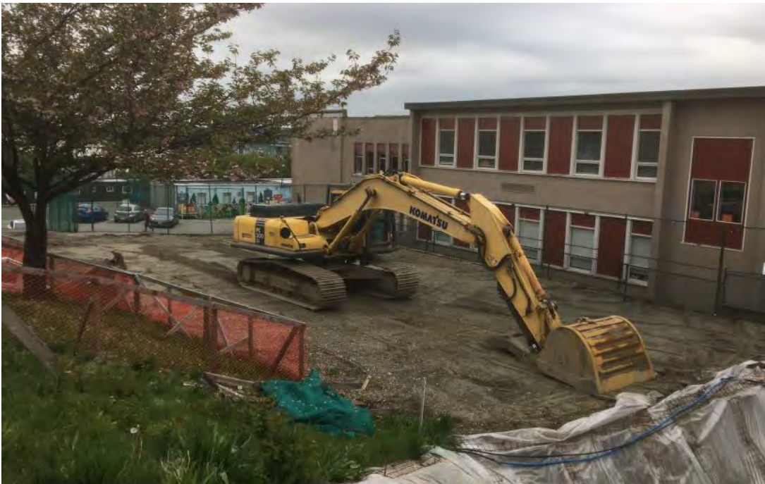
Excavation of former basketball court in preparation for underground services
