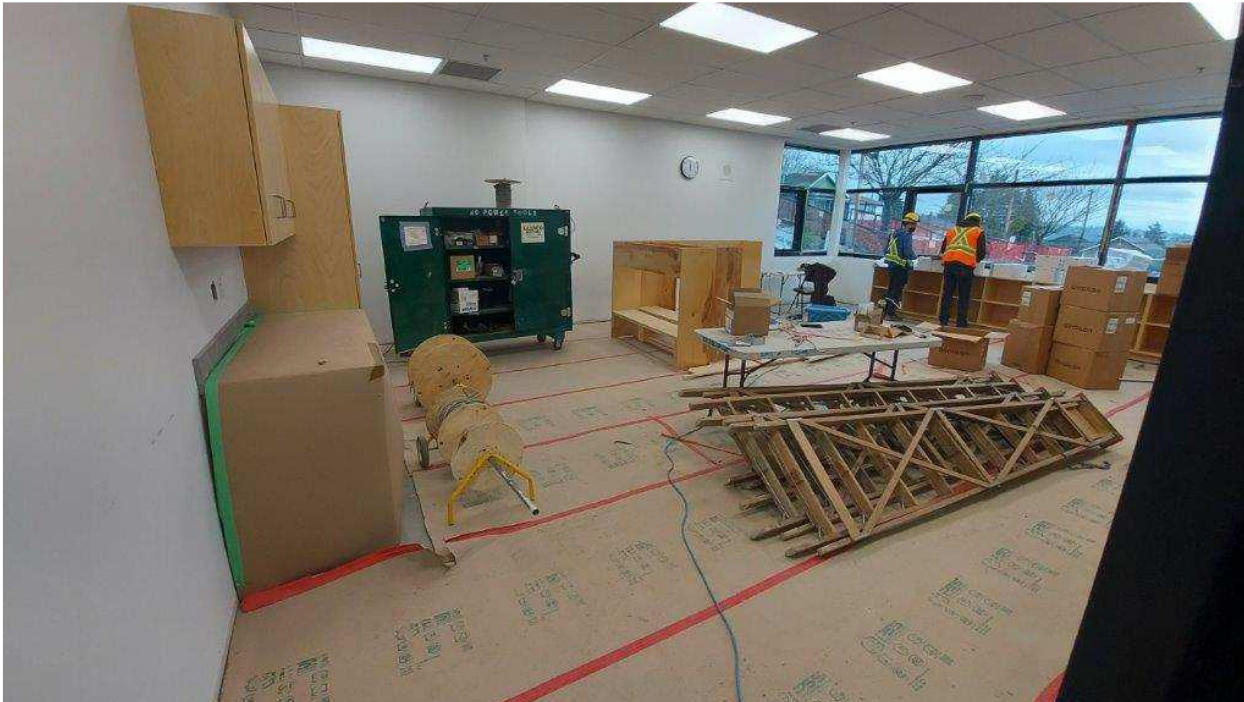
Classroom Millwork Installation (covering on floor to protect polished concrete)
