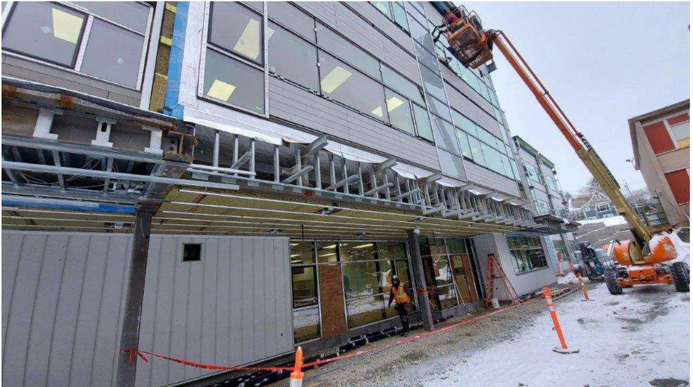
Exterior Cladding Progressing
