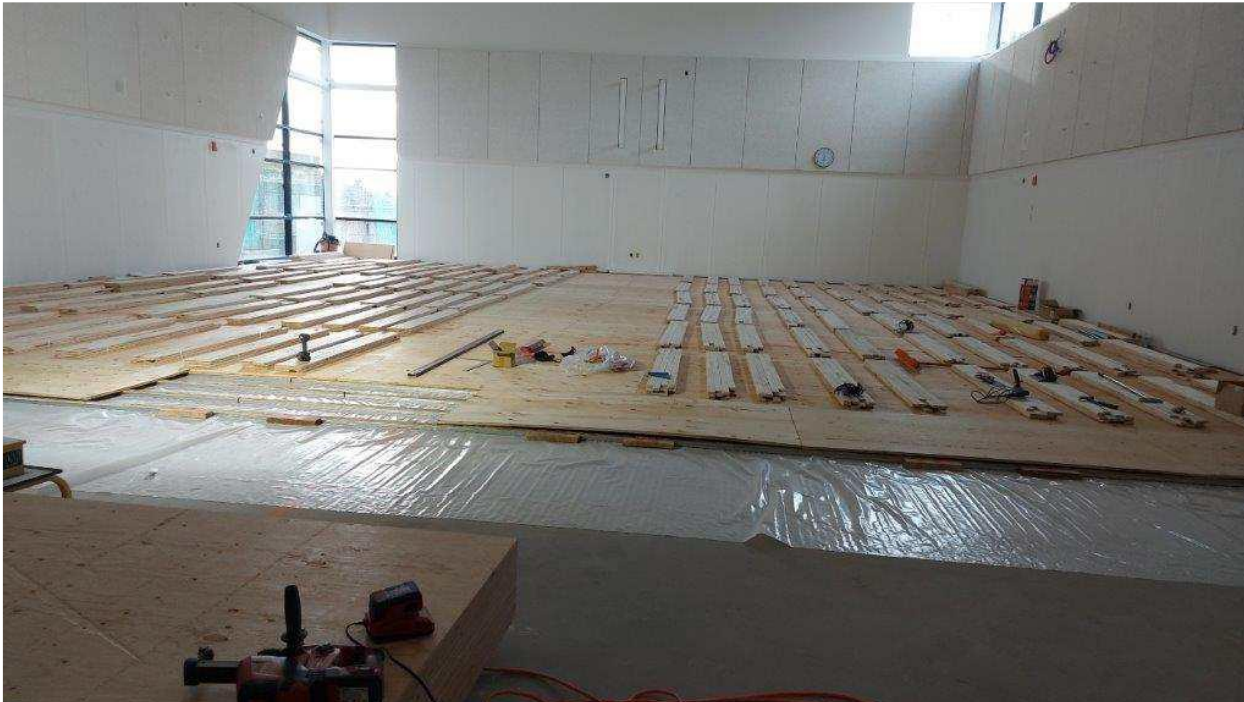
Gym Floor Progressing 1
