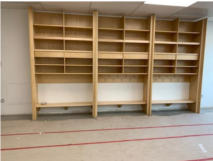
Classroom Millwork progressing
