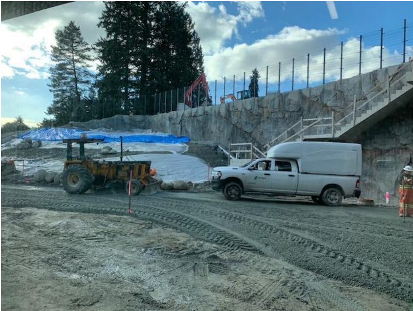
Exterior Courtyard Progressing
