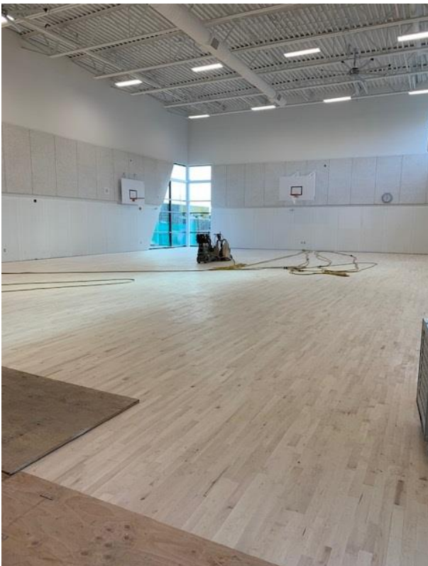
Gym Floor Installed with Sanding ongoing
