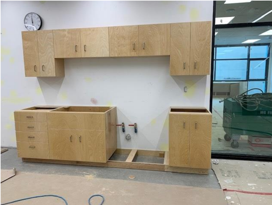
Collaborative Learning Space Millwork Installation
