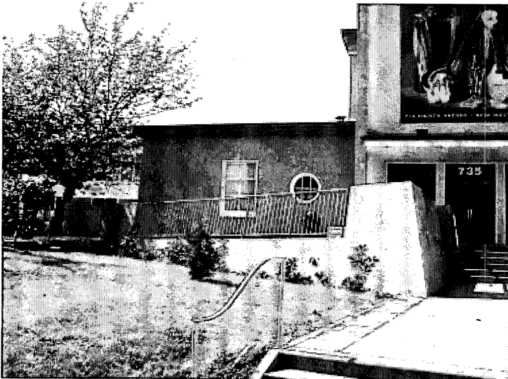
Photo 4: East View of Plaskett Gallery
