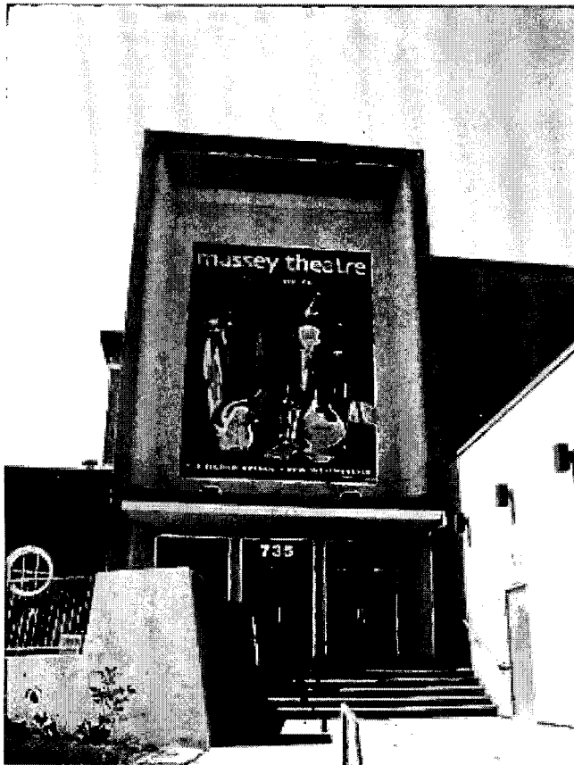
Photo 1: East Entry to Massey Theatre Description: East end of three storey lobby, concession and office area. Issue: Moment frame to be provided to restrain east end of block.
