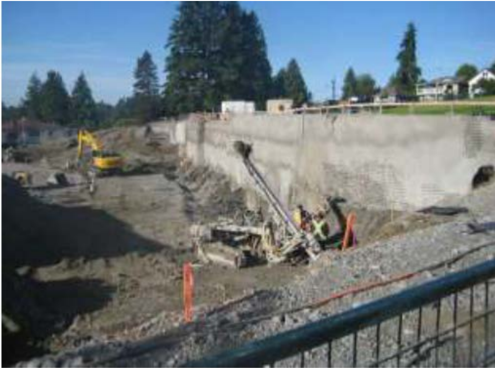
View of excavation extent and shotcrete wall
