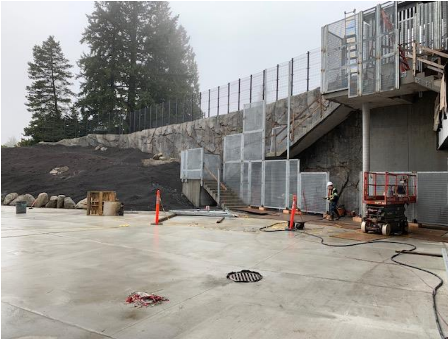
Installation of Stairway Railing nearing completion
