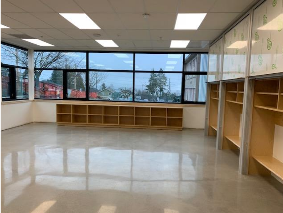
Classroom Millwork with Sliding White Boards Installed
