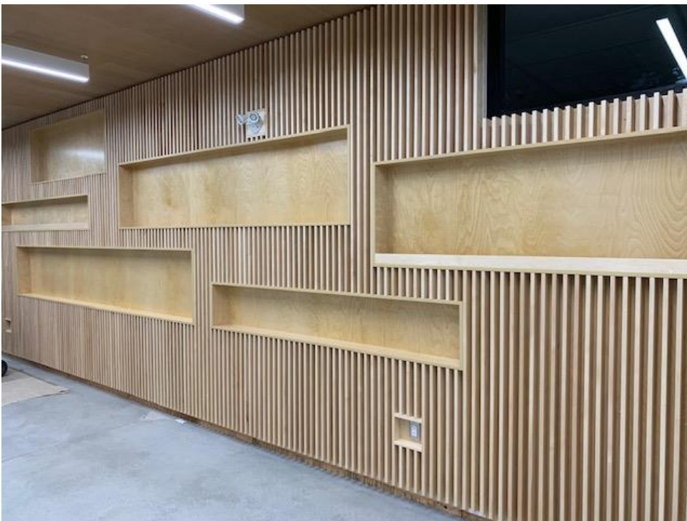
Entrance Feature Wall Nearing Completion
