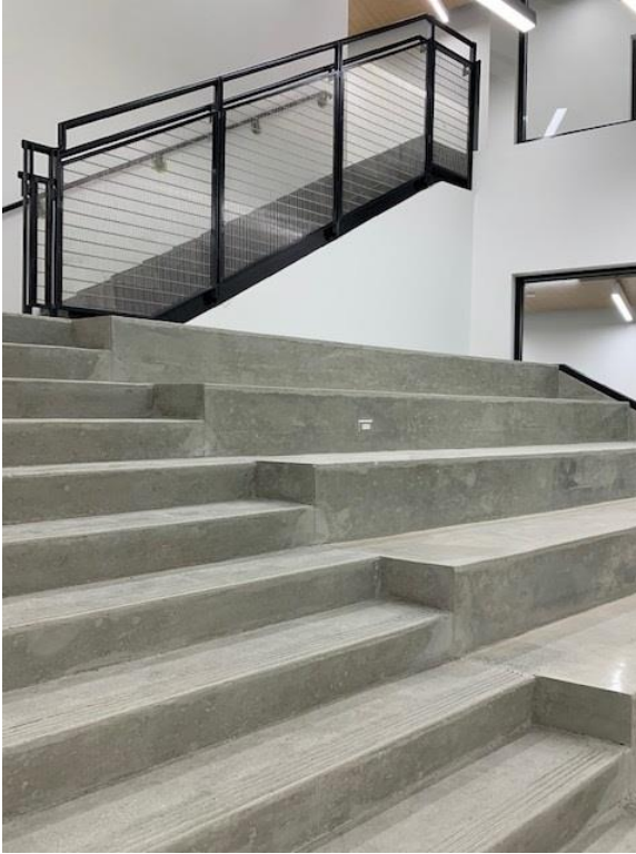
Stairs Complete with Glass installed
