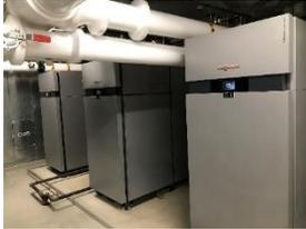
The new New Westminster Secondary School, with a student population of 1900 in a grade 9 to 12 setting, opened its doors in January of 2021 with a low-temperature hydronic system and efficient heat emitter solutions comprised of three large 3500 MBtu high efficiency condensing boilers to heat the 16390 sqm building. The condensing boilers must operate with return water temperatures below 38°C to maintain rated efficiency.
