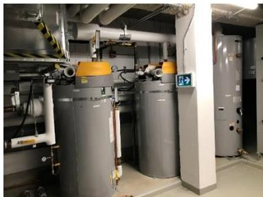
The modulating hot water heaters offer a 96% thermal efficiency, dramatically lowering energy use as they adjust firing rate to the specific demand with the large store tank and extra capacity storage tank. The system allows for monitoring remotely for diagnostic fault notifications and fault histories as well as controlling the set points and differential of the water
